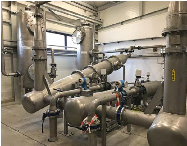
Photo 4. Biogas Purification System absorbing carbon dioxide
